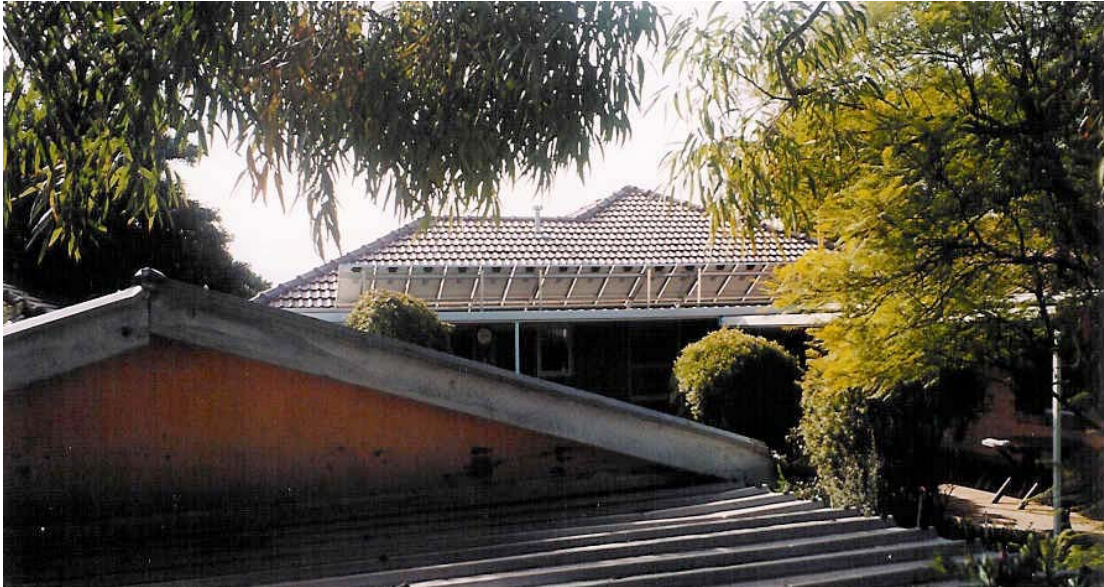
Figure 1: Mounting of solar panels on south side of house.
