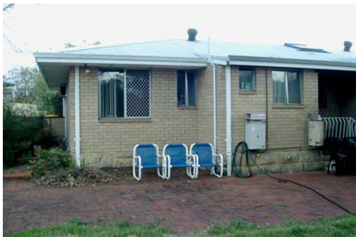
Original style of rear – typical 1960s home with bathroom to north.
